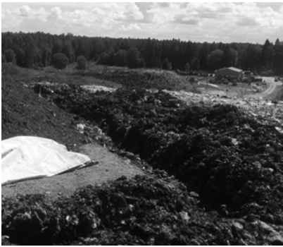
Fig. 2. Excavation of trenches
